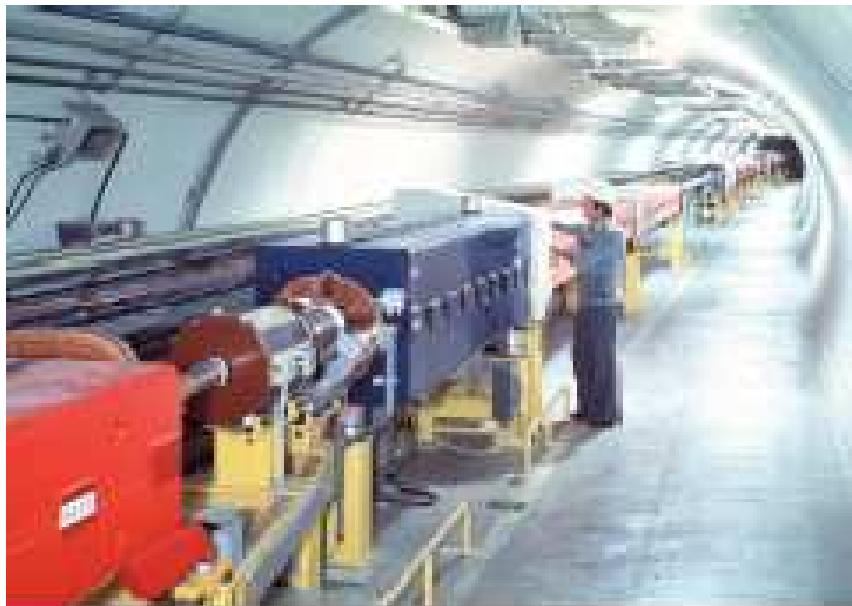
LEP Tunnel, 27 Km circumference
